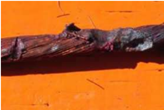
Arcing evidence: notching*
