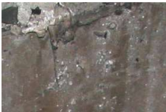
High energy splatter due to arcing*
